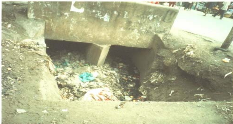
Picture 5. The picture above shows a drain in Nairobi blocked by plastic bags.
