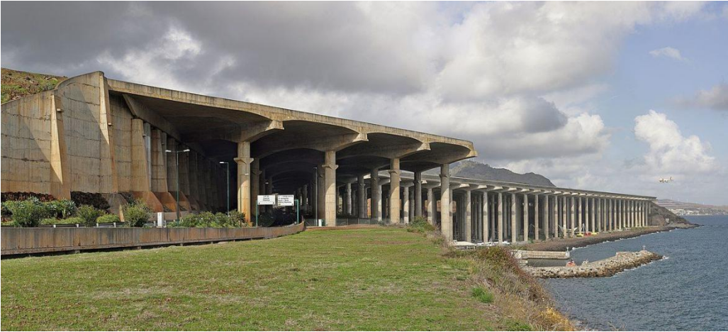
Figure.3. Supporting pillars under the airport runway extension(Madeira Airport 2023b)
