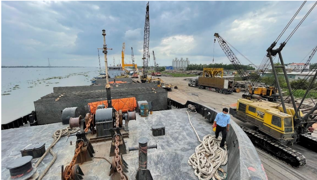
Figure 6. Weak infrastructure in the Mekong Delta
