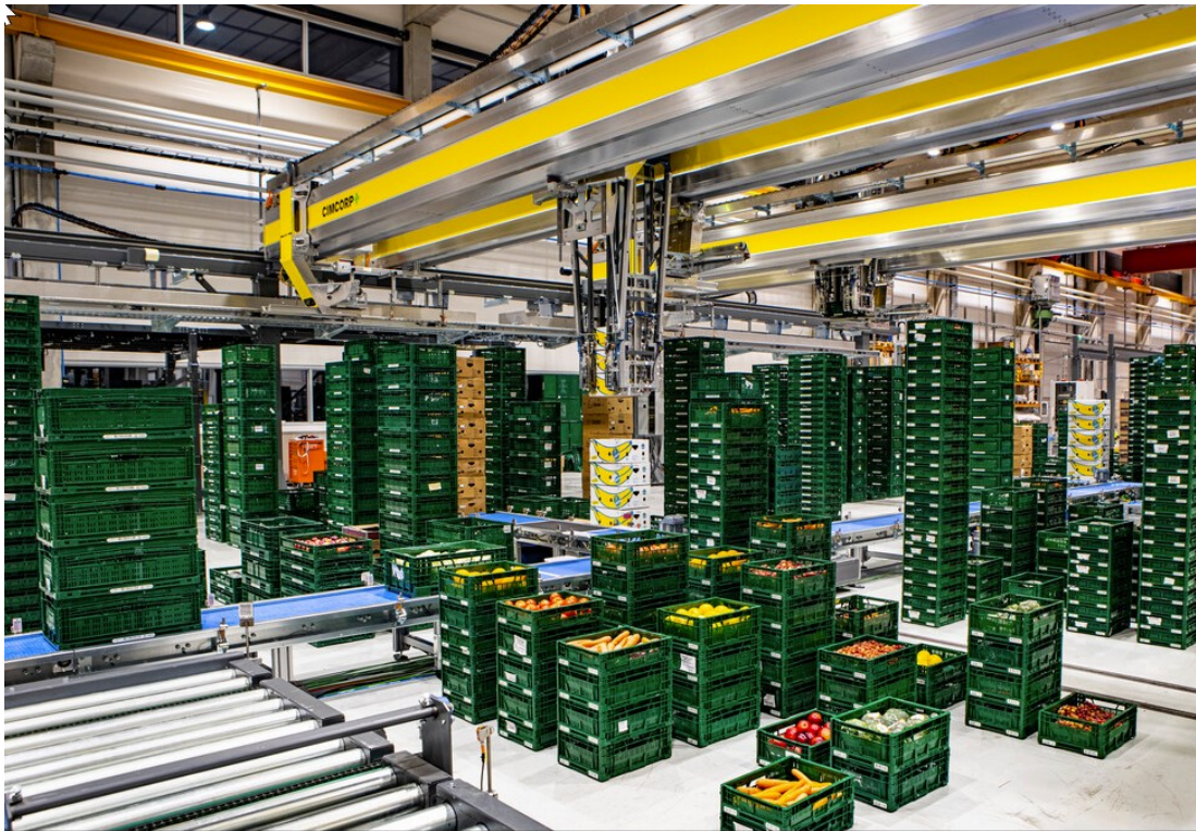
Picture 1. Cimcorp's customer company distribution centre (Cimcorp Media Collections)
