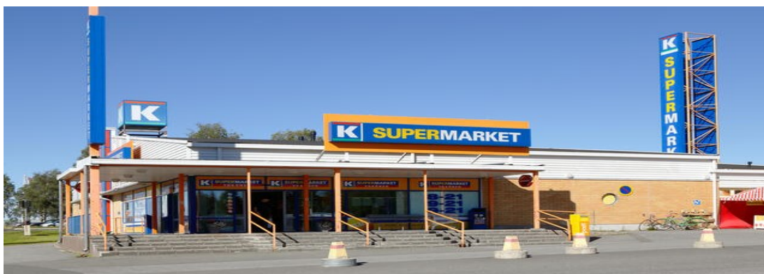
Figure 9. Kesko Supermarket Outlet.
