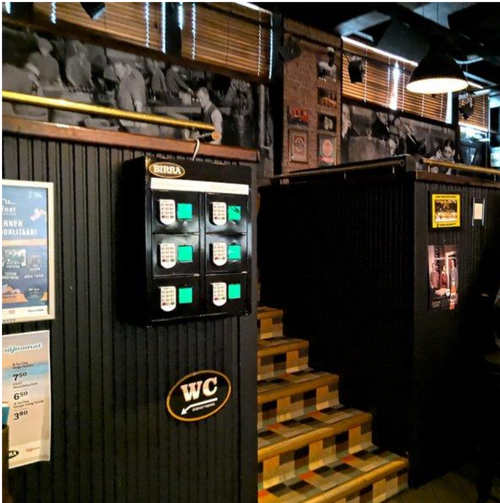
Figure 3 - Charging cabinet - https://vivotech.fi/tuote/vivotech-b6/
