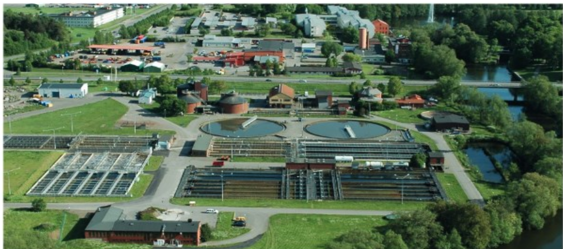
Wastewater treatment plant in Lindköping. Photo: Tekniska verken in Lindköping
