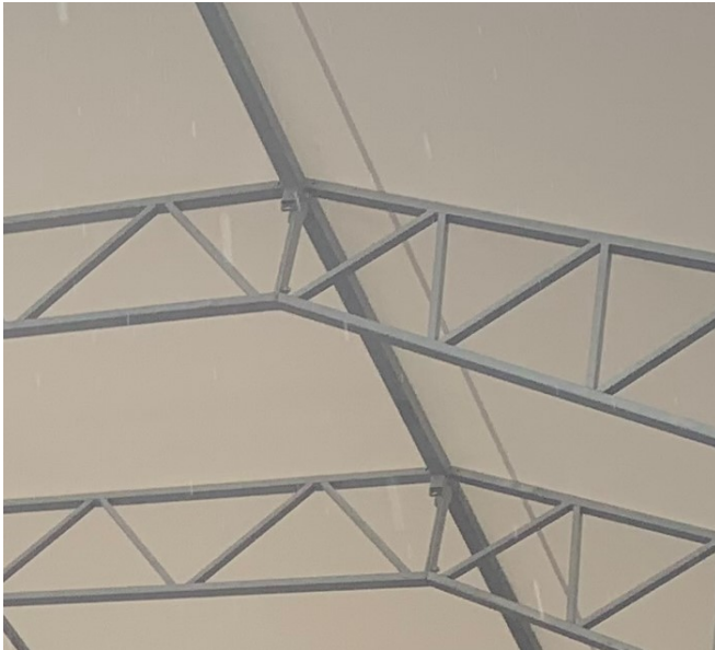
Figure 3. The purlin on the ridge of the roof and trusses.
