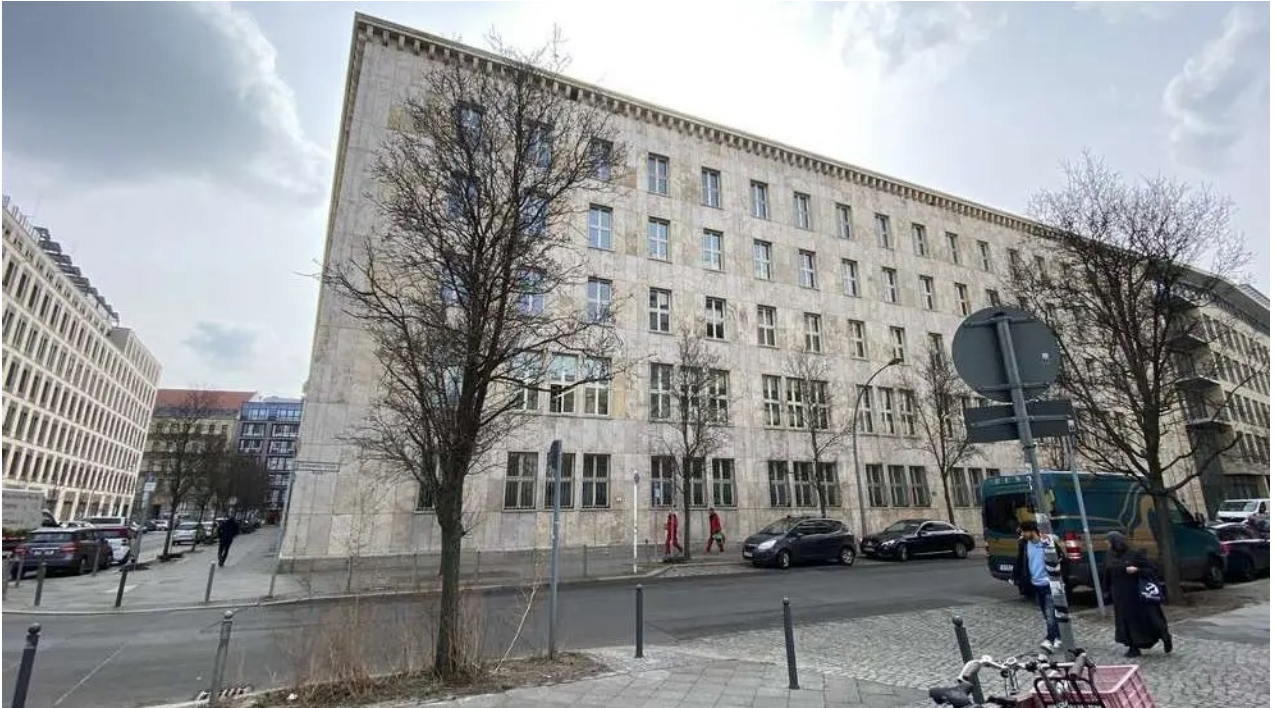
Fig. 11 Existing Conditions – Façade [88]
