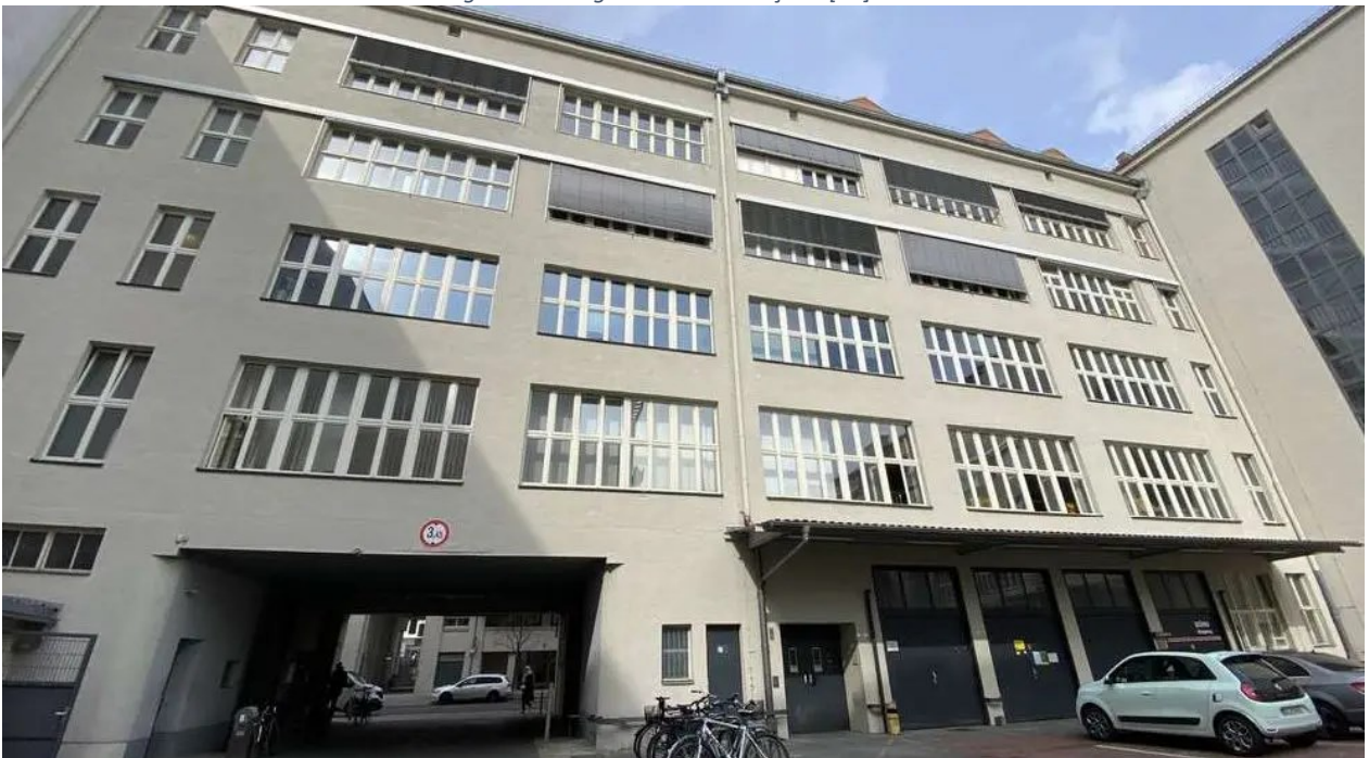
Fig. 12 Existing Conditions - Facade – Courtyard [88]
