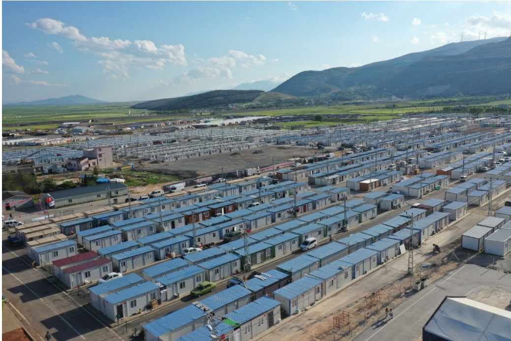
Figure 46: Container city set up in Nurdağı district of Gaziantep, Türkiye
