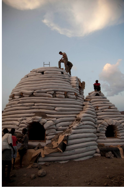
Figure 53: Super Adobe Vernacular house construction
