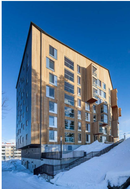
Figure 21: Puukuokka Apartment Building using CLT
