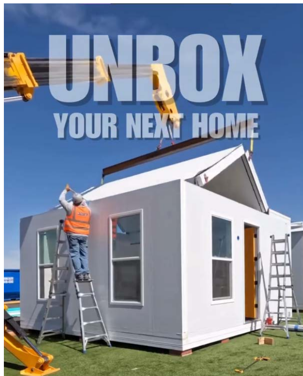
Figure 18: Boxabl housing unit assembly on site
