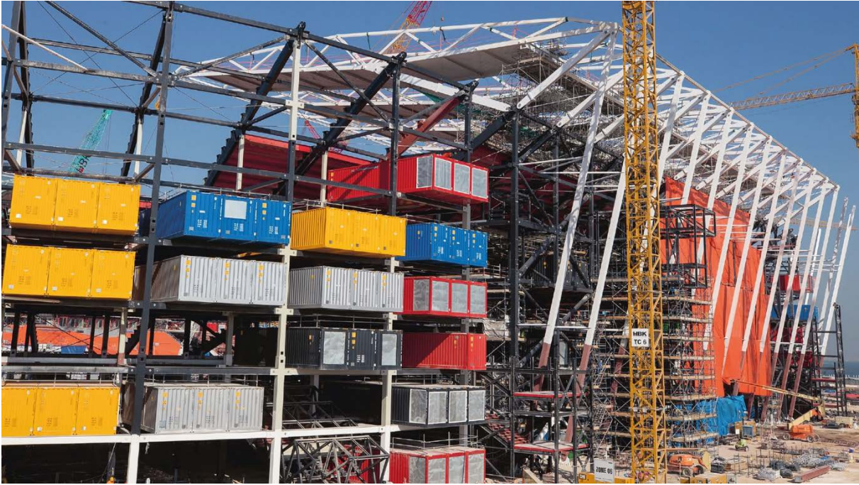
Figure 27: Stadium 974 using recycled shipping containers
