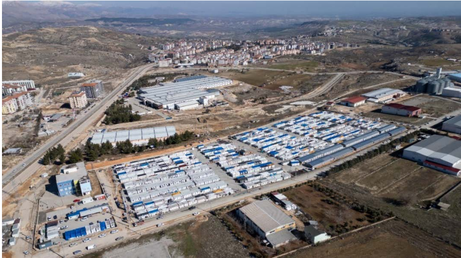
Figure 47: Container City in Besni, Turkey
