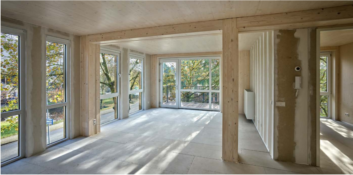
Figure 31: M'DAM project CLT construction inside view
