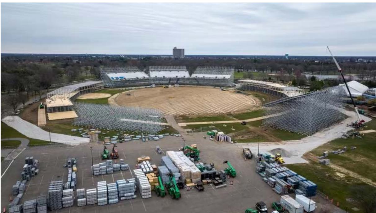
Figure 36: Construction in progress of T20 World Cup cricket stadium in March 2024
