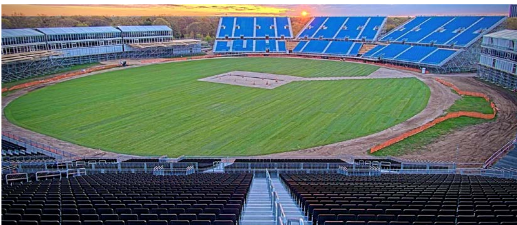
Figure 38: The completed stadium project
