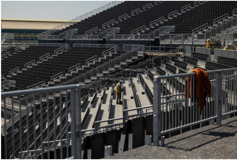
Figure 37: The Aluminium structure of the stadium in May 2024
