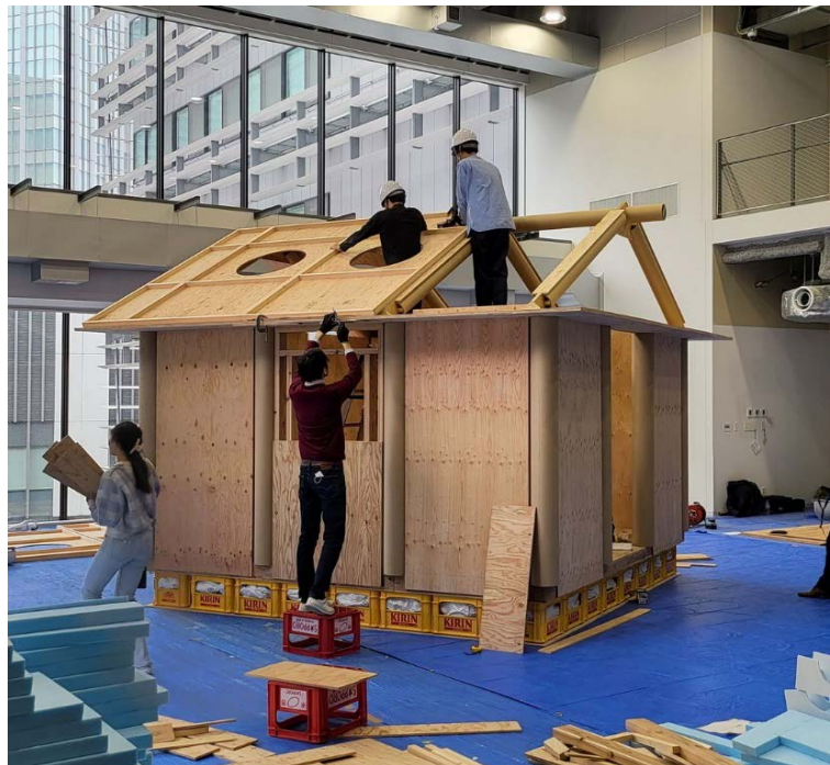
Figure 55: Paper Partition System (PPS) house prototype
