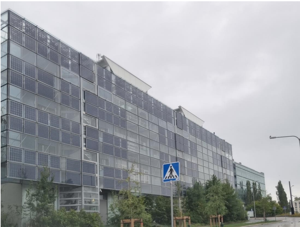
Fig. 6: A picture of BIPV on the exterior glazing of a building in Helsinki (Author, 2023)
