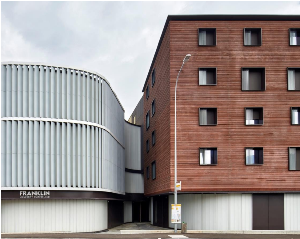
Fig. 17: An Exterior image of the BIPV shading system (Solarchitecture, 2024)
