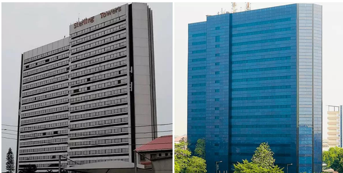
Fig. 1: A 6500m 2 BIPV installation by Onyx Solar on an office building in Lagos, Nigeria (Onyx Solar, n.d.)
