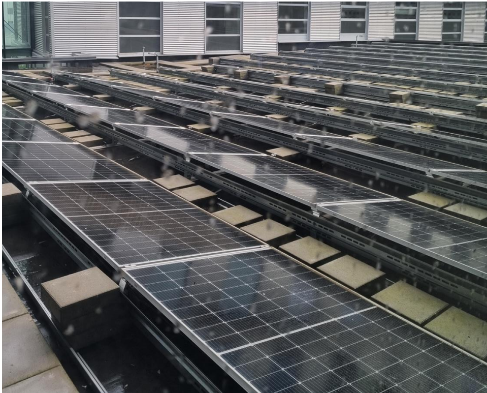
Fig. 4: A picture of a roof-top BAPV installation in a university building in Rotterdam (Author, 2024)
