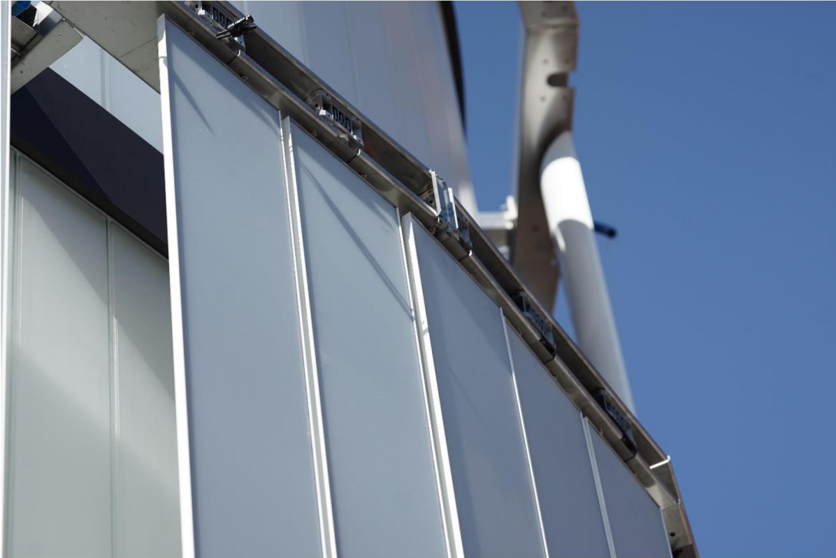
Fig. 19: A close-up view of the BIPV Slats on the façade (Corti, et al., 2022)
