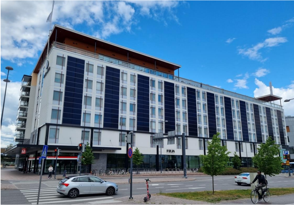
Fig. 5: A picture of opaque BIPV cladding integrated to the wall of a building in Helsinki (Author, 2023)
