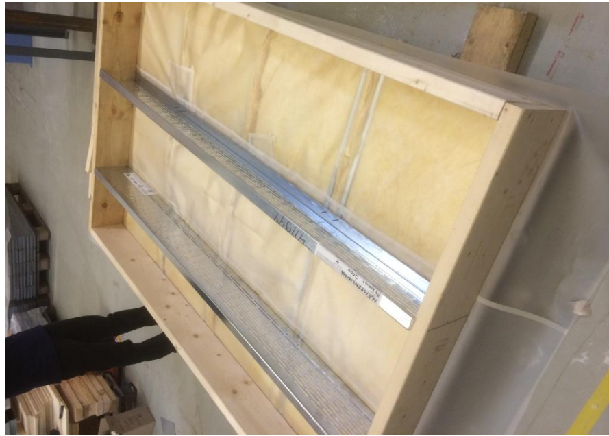
Figure 15 TERMO RANKA PURLINS and timber frame
