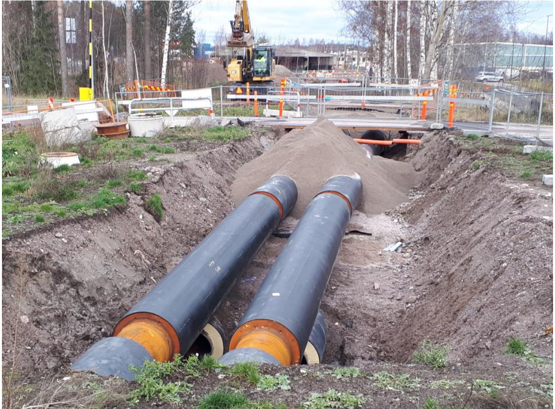
PICTURE 4. Bonded pipes (Jari Randell)
