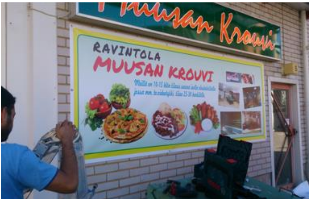
Figure 15: Installing Plastic Sign board
