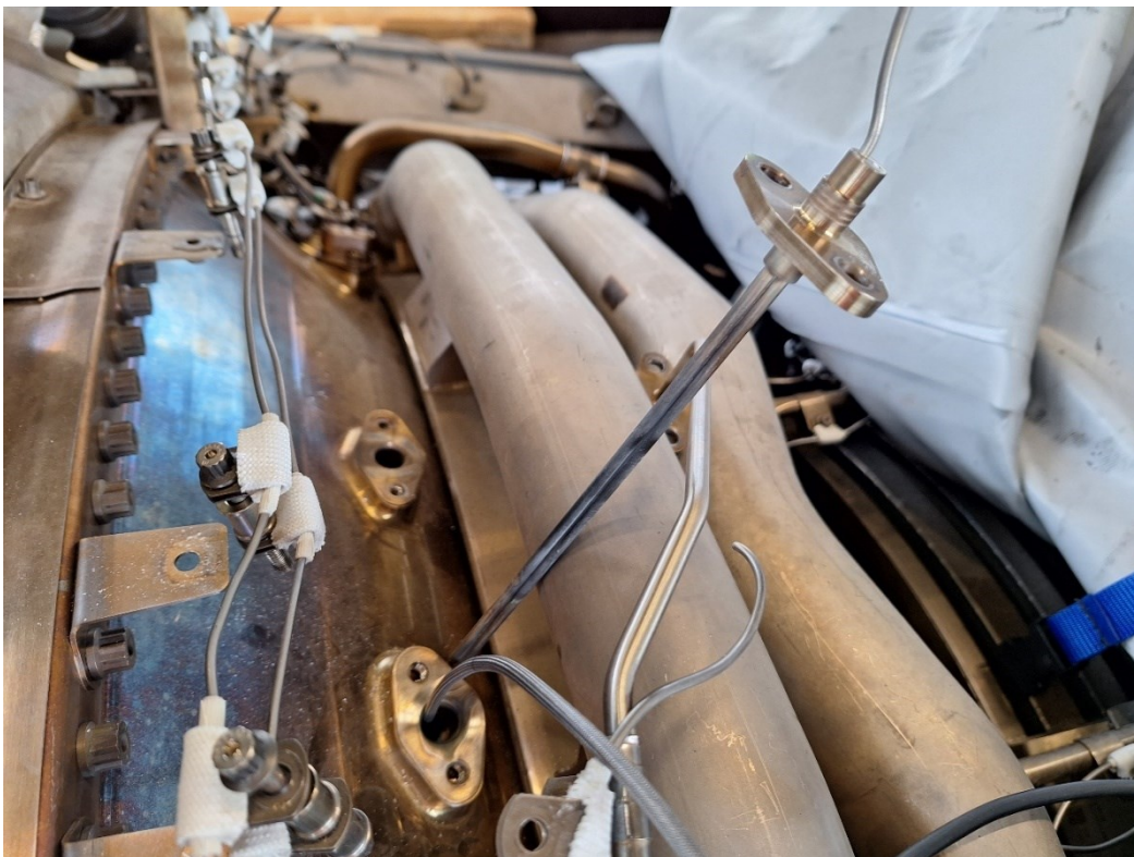
Figure 11. Borescope Insertion Location
