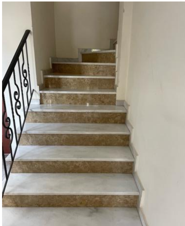
Photo 2. A staircase entrance in block flats
