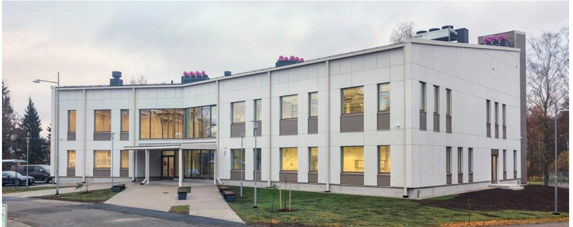
Figure 8. The HAMK Smart Bio building in Autumn 2024
