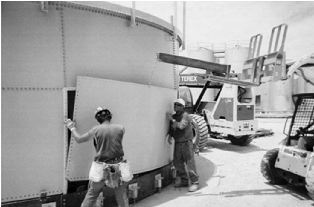
Figure 7. Installation of Lap joints (Buys, 2024)
