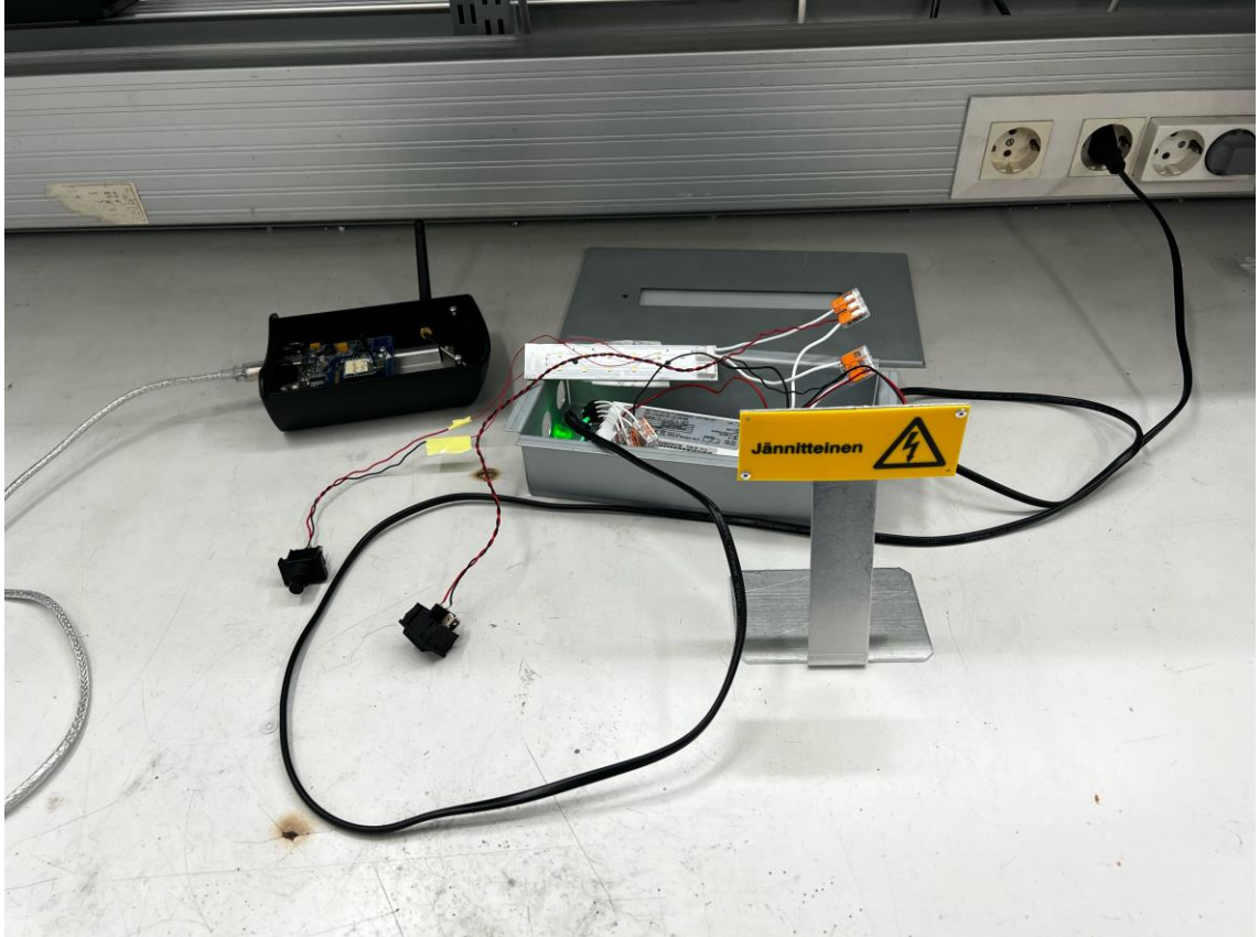
Figure 8. A staged DUT with its casing and a “live voltage” sign next to it.
