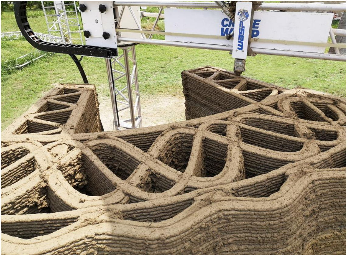
Figure 15:Tecla house raw earth printing (Copyright © Mario Cucinella Architects and WASP, 2021). Photo by Iago Corazza.
