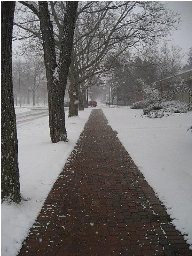
Figure 7. A heated sidewalk in Holland, Michigan [22]
