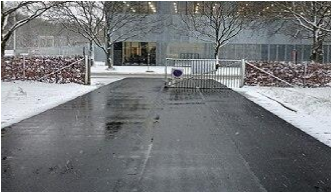
Figure 9. System installed snowless, Brandenburg, Germany [22]
