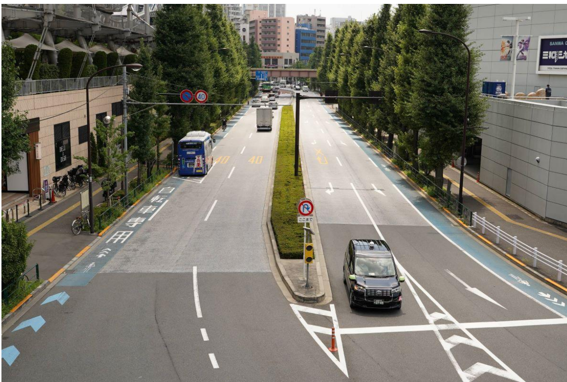
Figure 7. Roads paved with temperature suppressing pavement, July 18, 2024 in Bunkyo Ward, Tokyo (Sankei Shimbun 2024)
