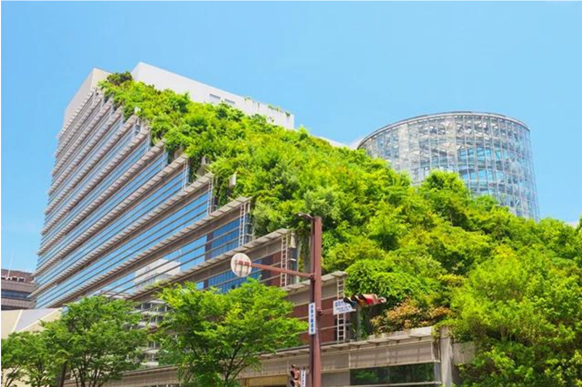
Figure 6. View of the Acros Fukuoka Building (Yyama 2015)
