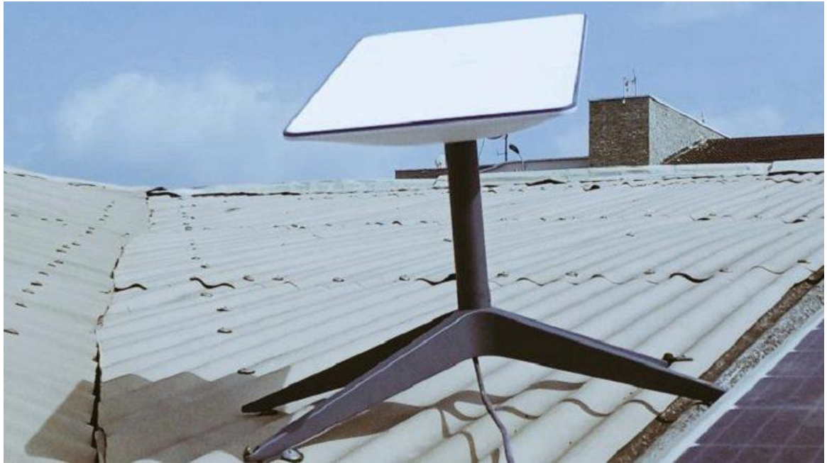
Figure 2. Installed starlink equipment at test location
