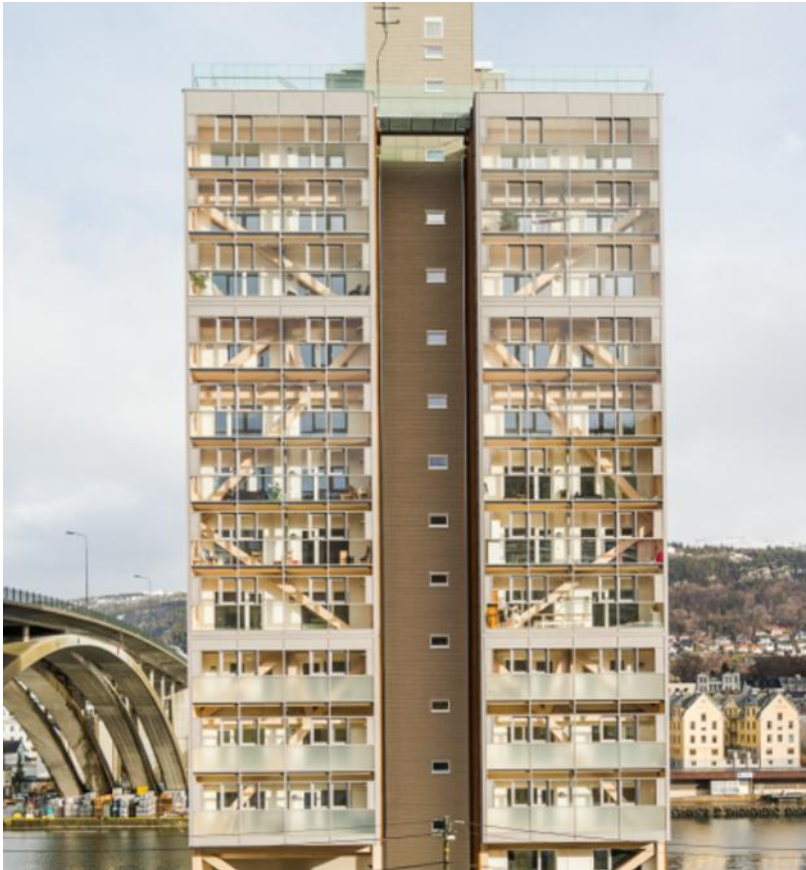
Figure 6. Treet tower in Norway (Woodhouse, 2025)
