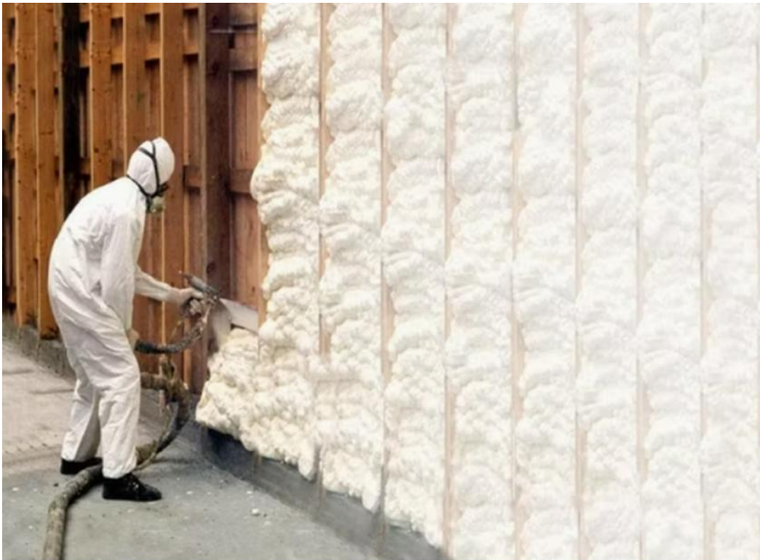
Figure 19. Polyurethane spray foam (Gnsgroup, 2025)
