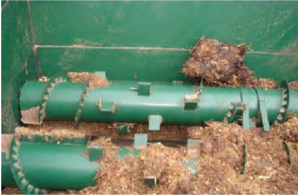
Figure 6. Co-substrate feeding system [13]
