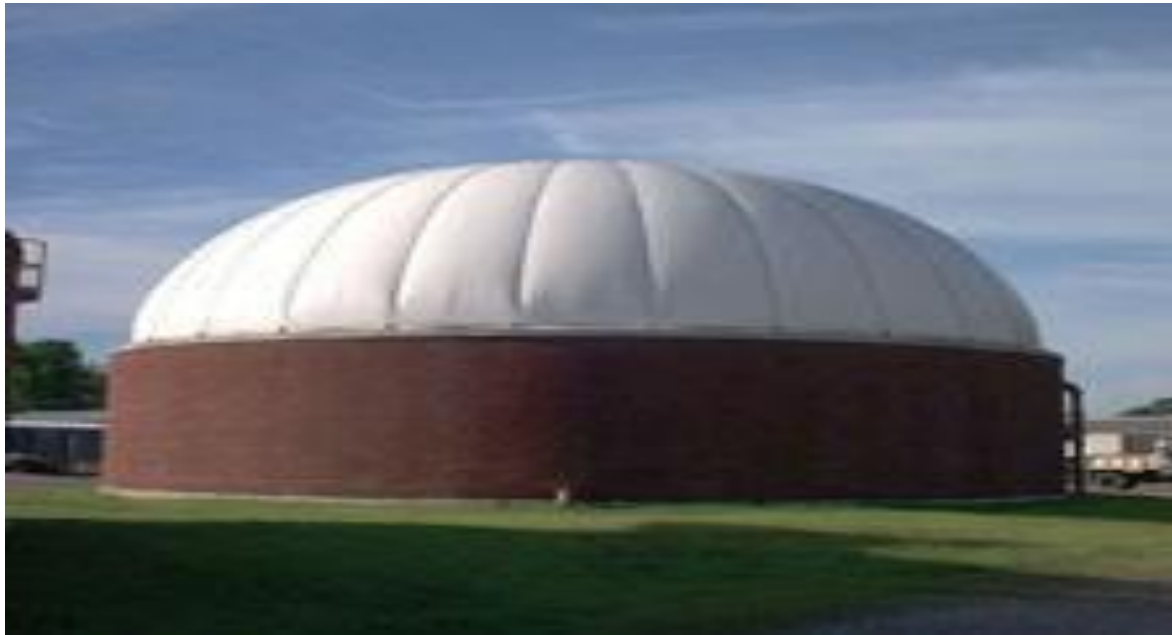
Figure 13. Internal biogas storage [17]
