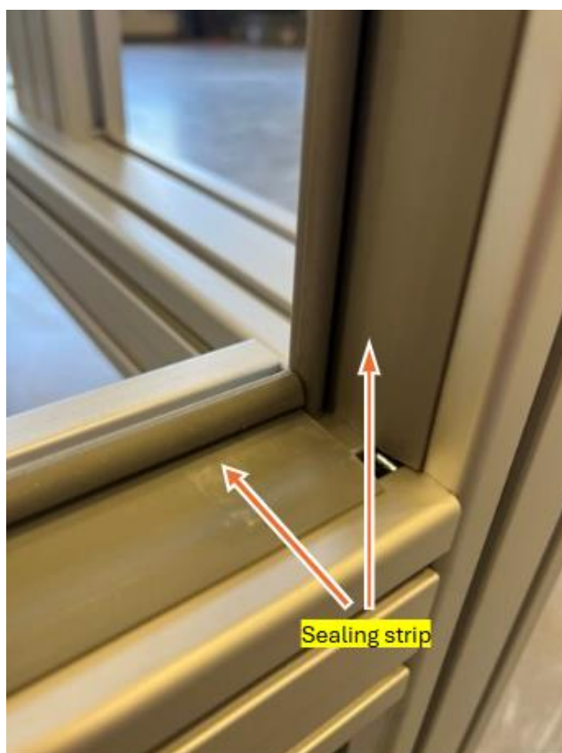
Figure 44. Close-up of the installed sealing strip for the door.
