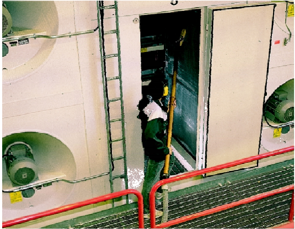
Figure 7. The wire screen frames are cleaned with vacuum cleaner.
