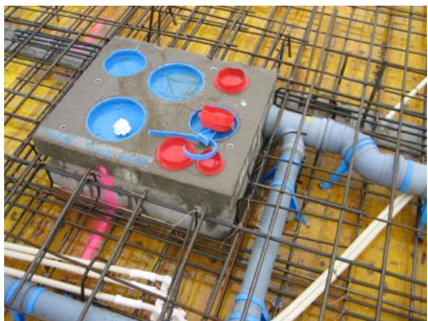
Img. 404. Head of a technical element to be fixed inside the cast concrete
