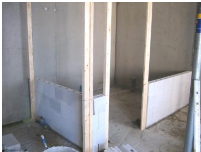
Img. 413. Assembly of a small format block wall
