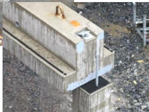
Img. 344. Detail of a beam resting over the column
