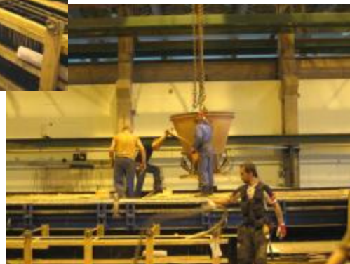
Img. 373. Casting concrete
