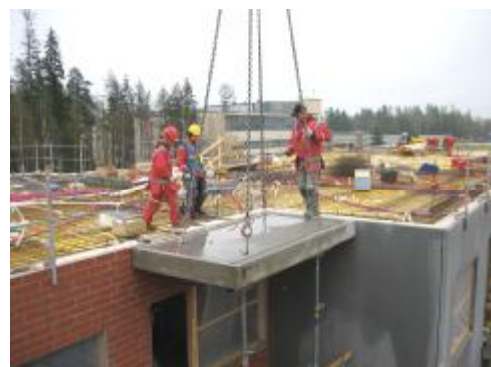
Img. 380 - 383. Sequence of the placement Of a balcony element
