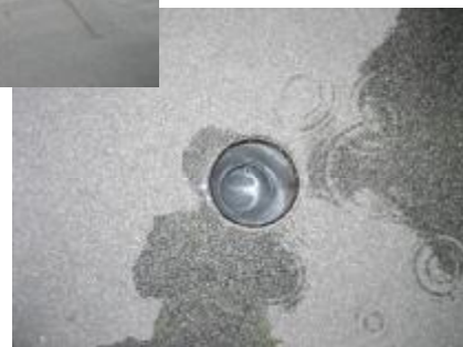
Img. 427. Placed drain
