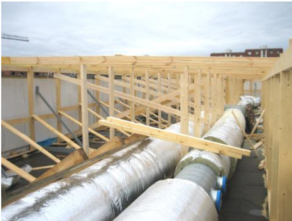
Img. 420. Sight of the timber system
