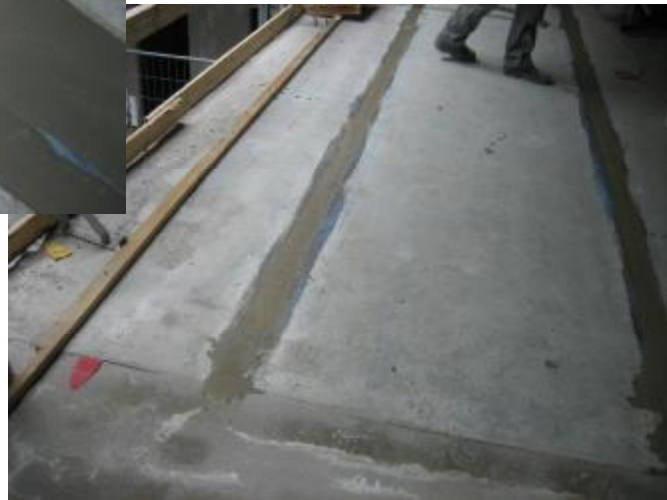
Img. 354. Surface of a beam covered with the cement liquid mixture
