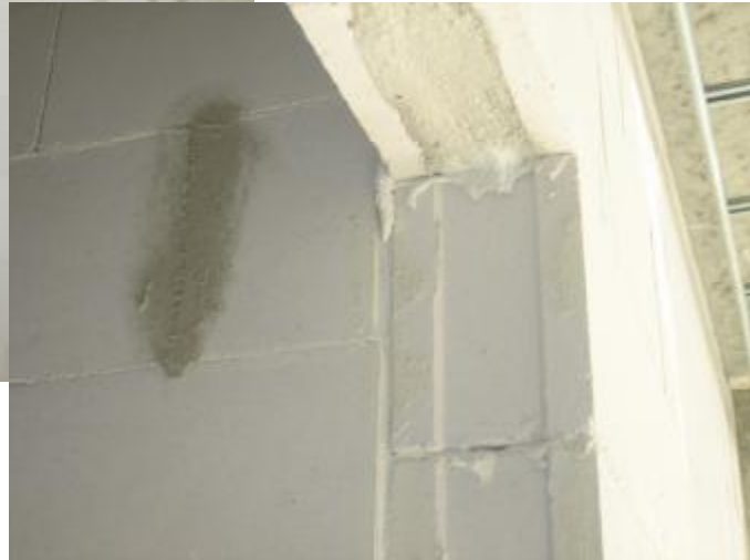
Img. 412. Detail of the lintel
