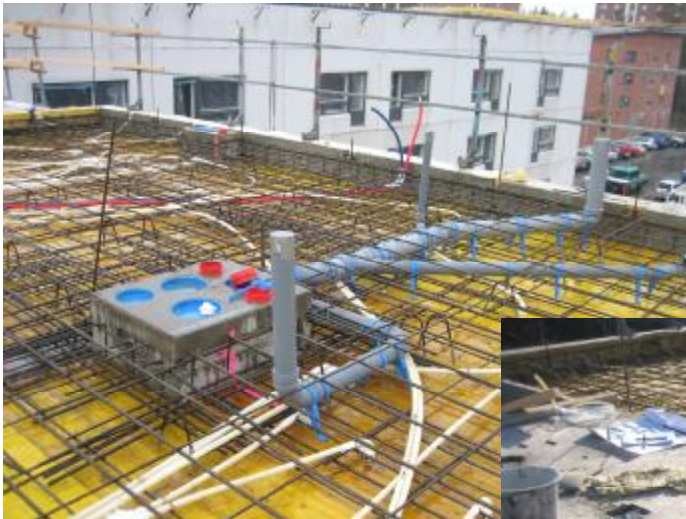
Img. 506, 507. Heads of technical elements, connected with the drainage installation
