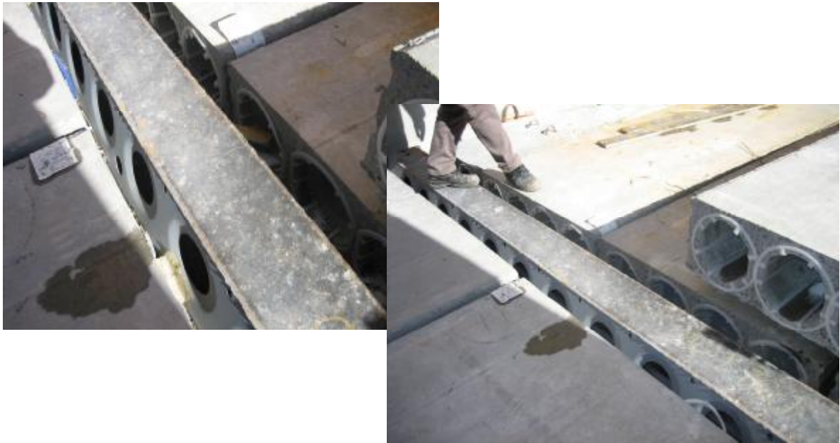
Img. 348, 349. Views of the metal beam system
