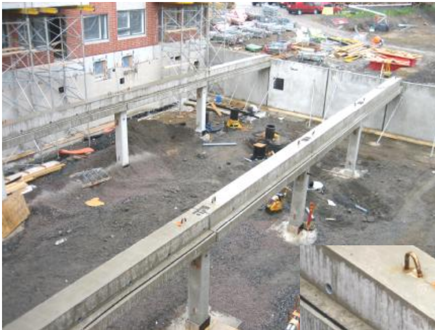
Img. 343. Set of beams of the slab system
