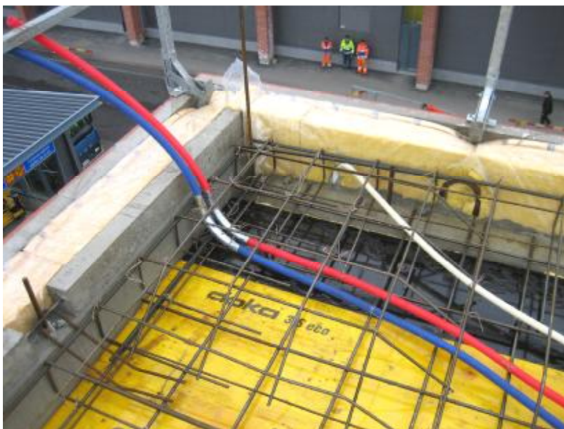
Img. 503. Connection of the cast concrete slab and the wall elements
