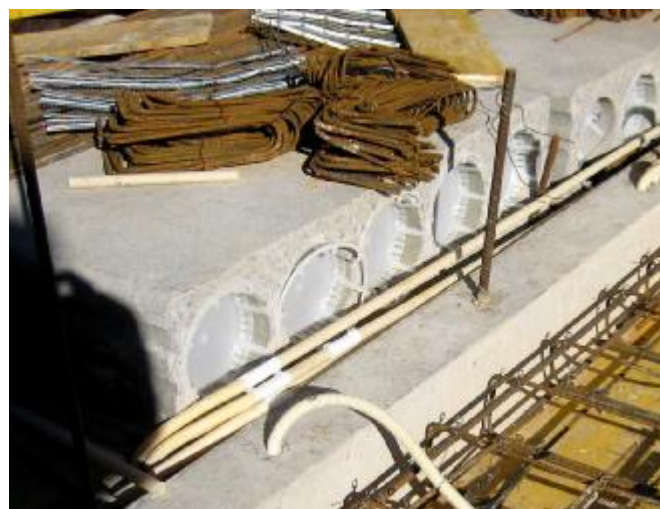
Img. 356. Plastic tops for concrete at the end of a slab panel
