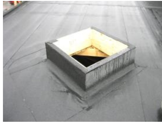
Img. 423. Joint of the roof with a wall Img. 424. Joint of the roof with a an access hatch
