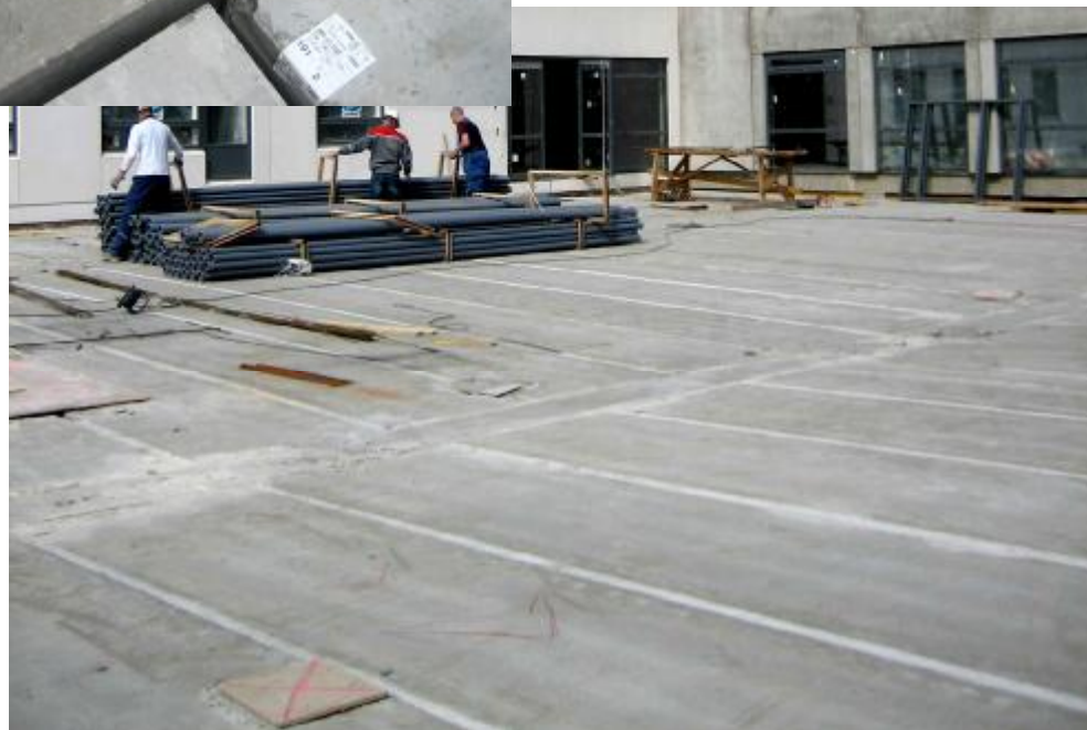
Img. 346. Aspect of slab system after filling the joints with concrete
