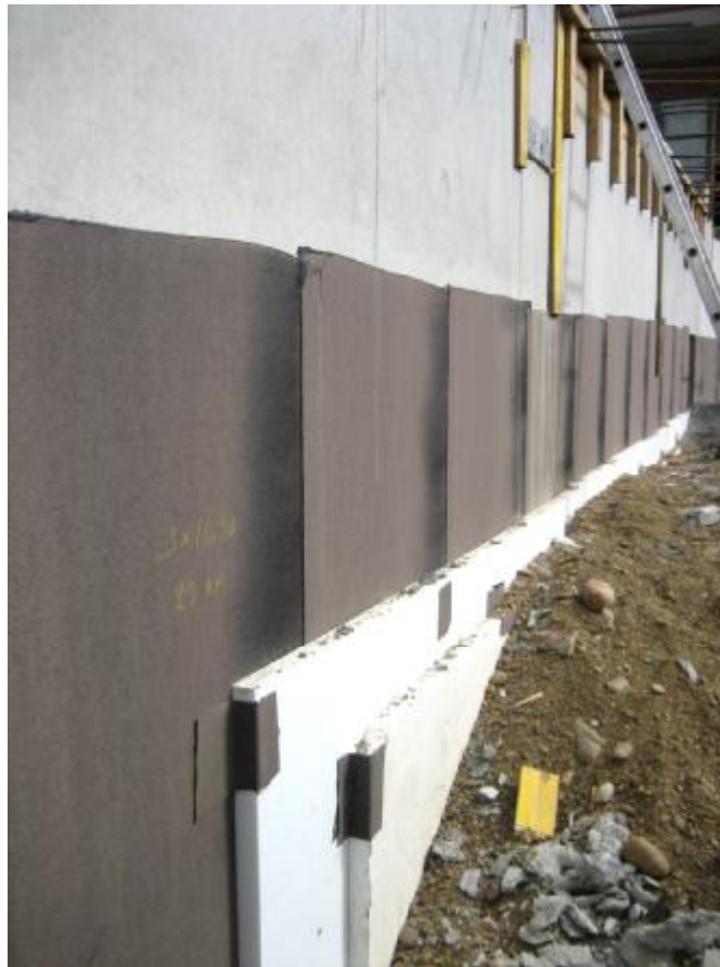
Img. 313. Exterior side of a basement wall of the building
