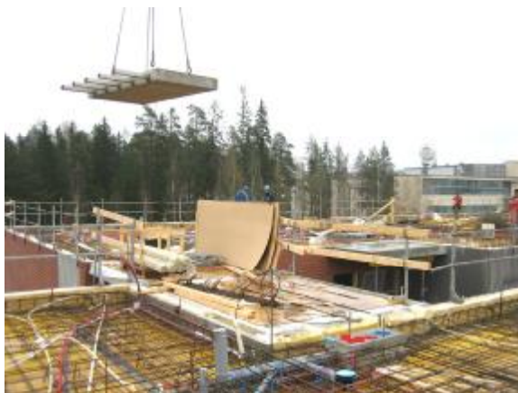
Img. 379. Hoisted of a balcony element
