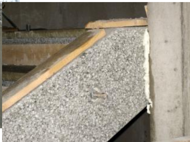
Img. 398. Lateral joint
