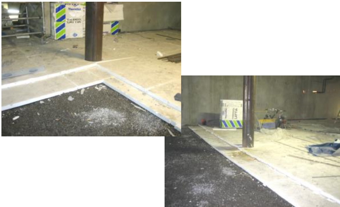
Img. 314, 315. Sight of the gravel layer and the insulation layer
