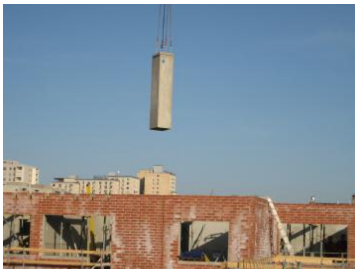
Img. 402. A technical element hoisted by the crane
