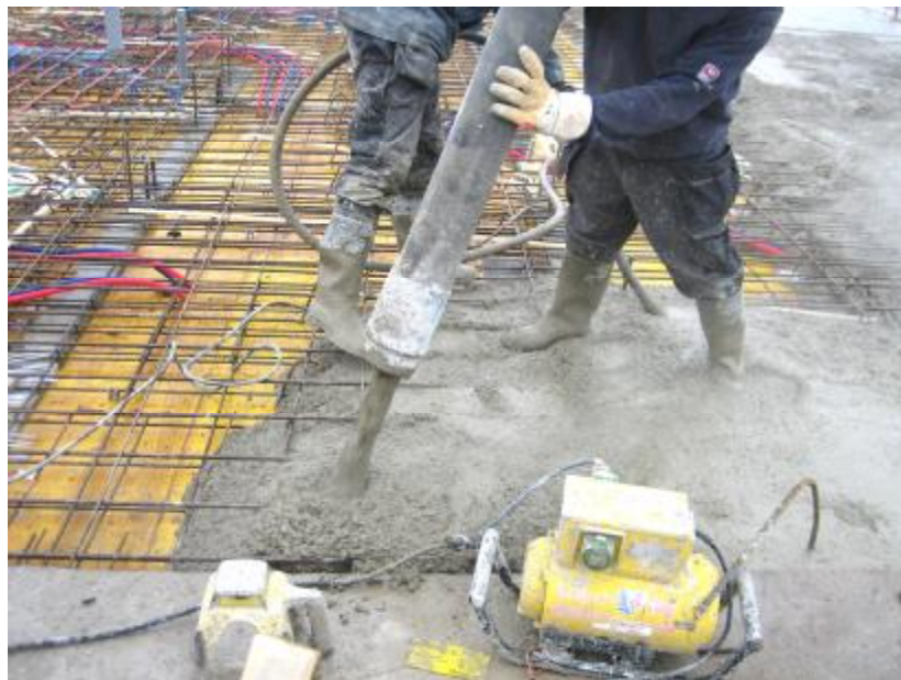
Img. 312. Casting concrete
