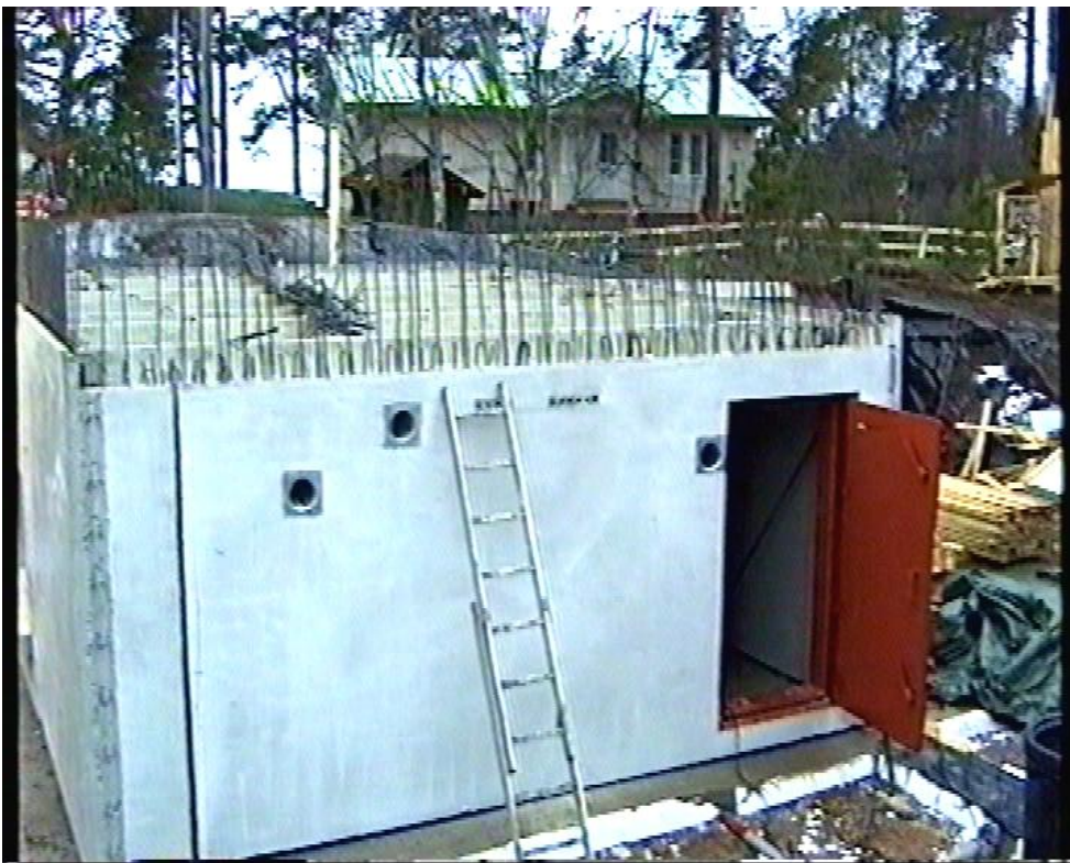
Img. 304. Image of a bomb shelter under construction
