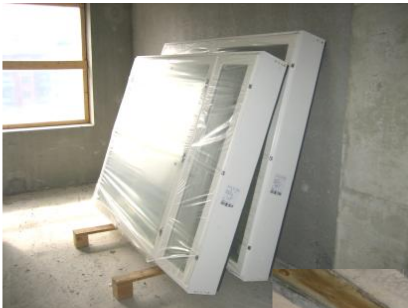
Img. 429. Windows ready for its placement
