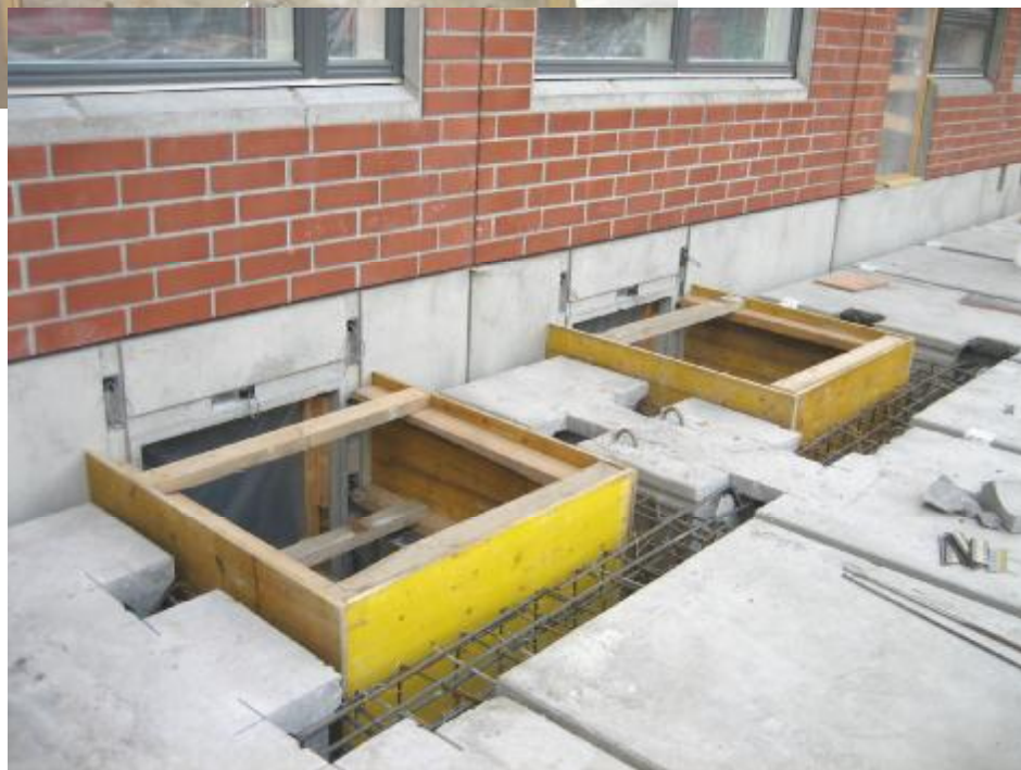
Img. 309. The emergency exits of the bomb shelters, goes outside through holes like those in the slab.
