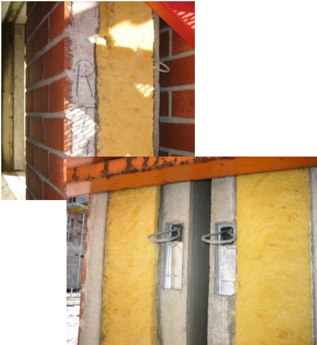
Img. 321, 322. Sections of prefabricated panels of front
