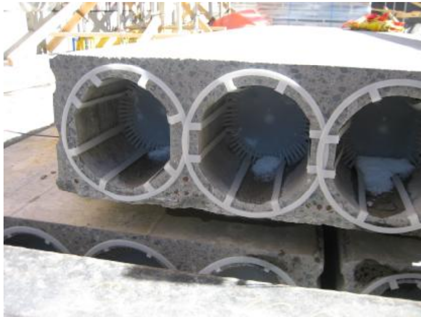
Img. 357. Big depth plastic tops for concrete. The ends of these elements will bear a big stress
