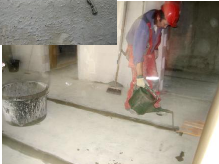
Img. 353. Workman spreading the liquid cement mixture
