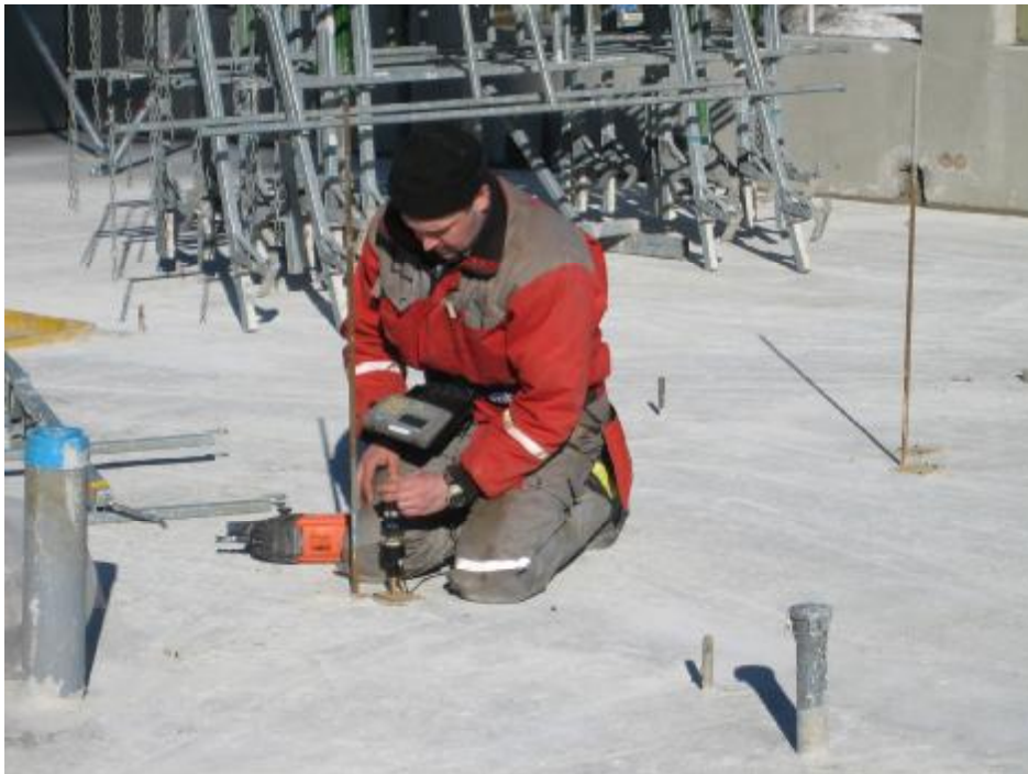
Img. 526. Surveyor and the remote control of the total station with a radiolink
