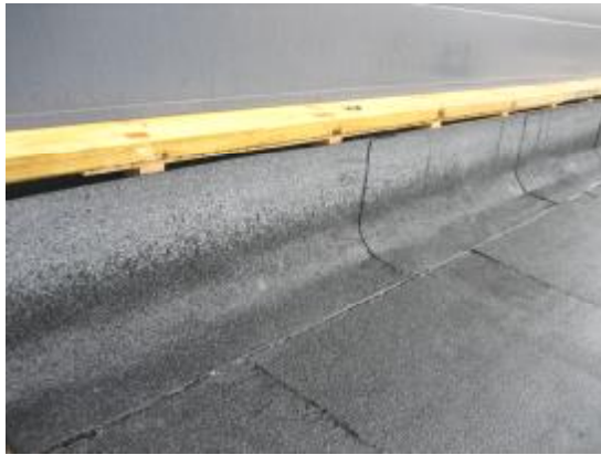
Img. 423. Joint of the roof with a wall Img. 424. Joint of the roof with a an access hatch
