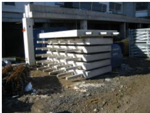
Img. 376. Stock of balcony slabs
