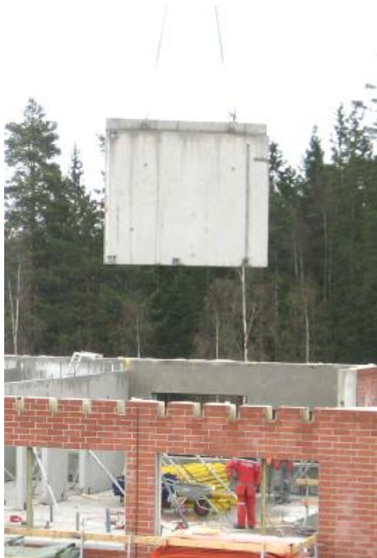
Img. 311. Wall element carried by the crane in the building site
