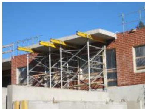
Img. 377. Temporary support for a balcony slab
