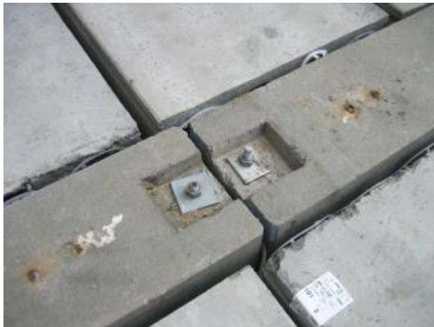
Img. 345. The ends of the beams ready For the concrete casting
