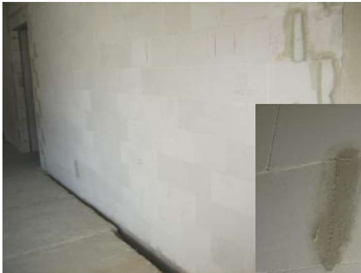
Img. 411. General aspect of the thick lime sand blocks wall
