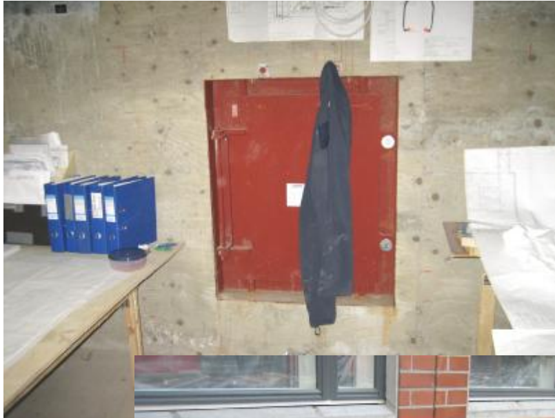
Img. 308. One of the emergency exits of of the bomb shelter
