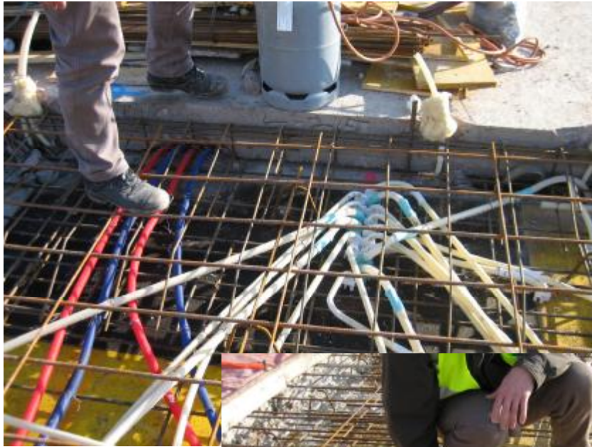
Img. 509, 510. Pipes for the electrical installation and the plumbing installation
