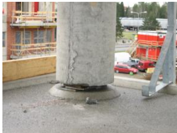
Img. 339. Column supported on sheets
