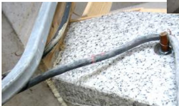
Img. 397. Low side of the upper joint
