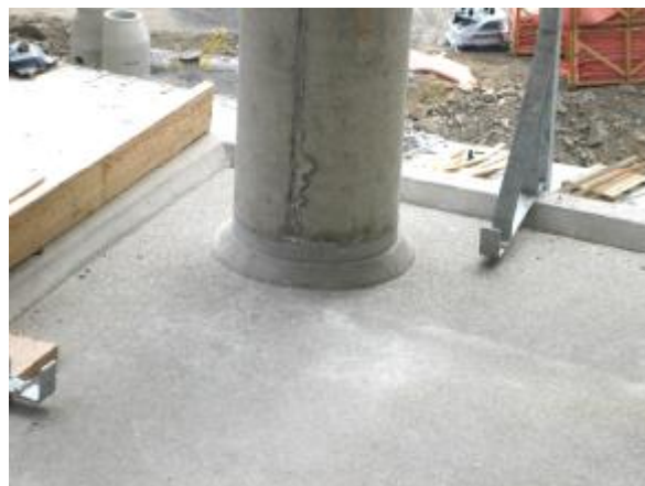
Img. 340. Final cement sand mixture recovered
