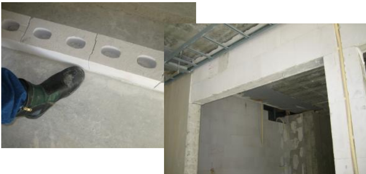
Img. 409. Sight of the thickness of the wall
