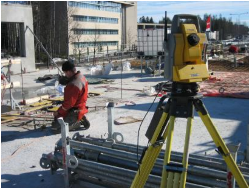
Img. 524. The surveyor and his total station equipment
