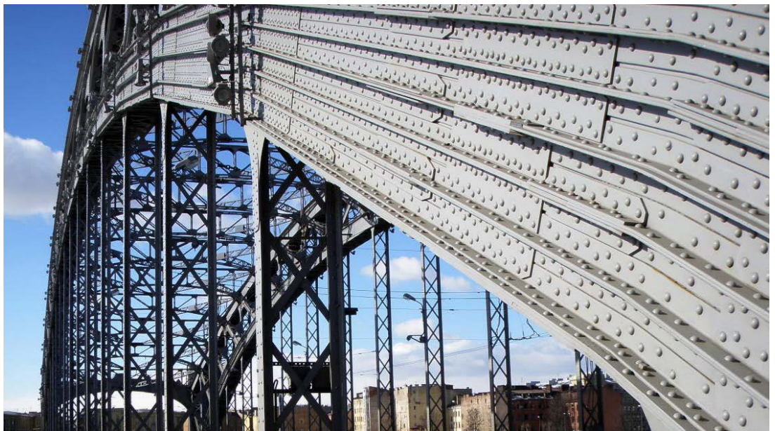
Figure 2.4. Rivet connections of the steel bridge constructions
