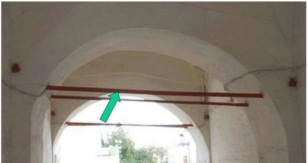
Figure 2.1. The tie in a brick arch
