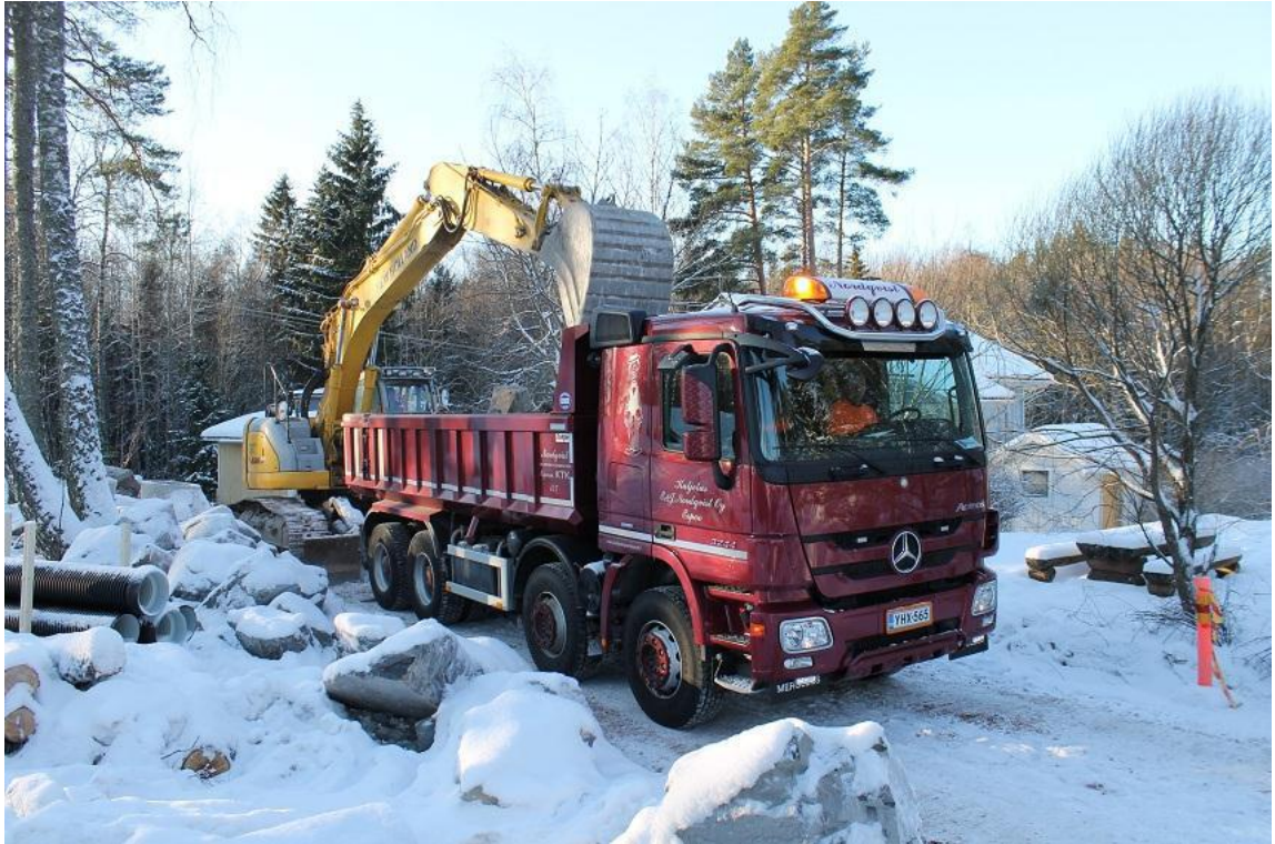
Figure 4. Standard 4-axle earthmoving truck being loaded under an excavator.
