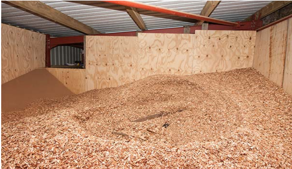
Figure 10. Wood chip silo with sloping floor in Glasgow UK. (AC Gold Energy, 2015).
