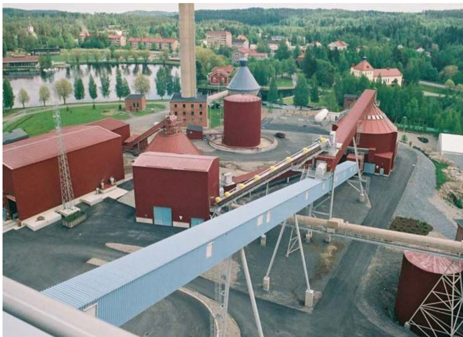
Figure 9. Fuel receiving and handling system in Jämsänkoski power plant. (Hakkila 2004, 50).
