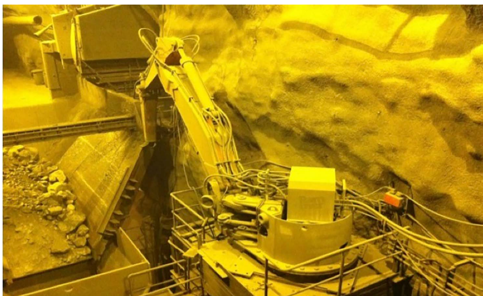
Picture 3. Underground hydraulic manipulator.
