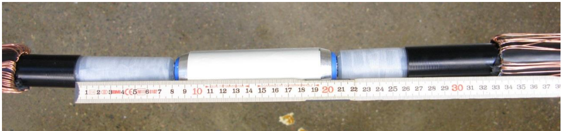
Figure 29. Too short insulation screen shaving on the right side of the connector.
