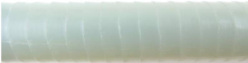
Figure 22. The shaving marks found from a cable joint that was removed from the distribution network.
