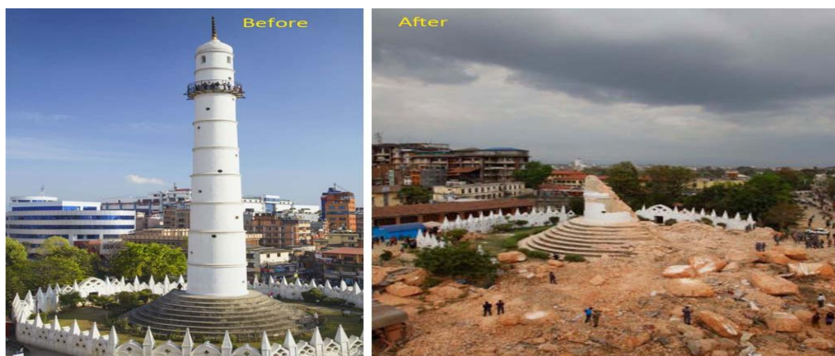
Picture 1; Picture of Dharahara before and after an earthquake
