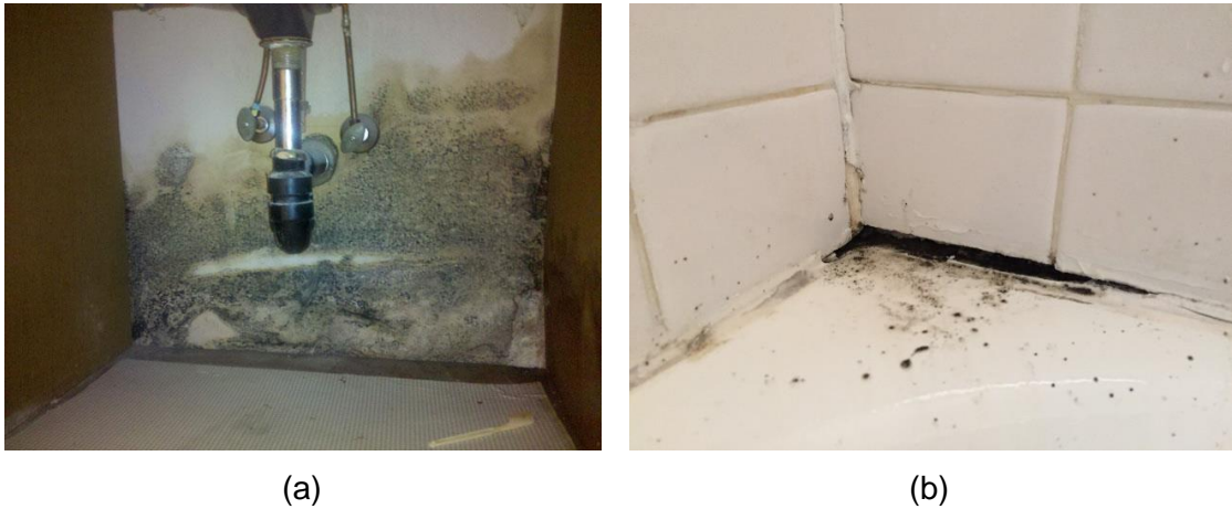
Figure 2.2 Figure (a) and (b) showing growth of mold in damp places (Paragon, ei pvm) , (Stephen, 2015)
