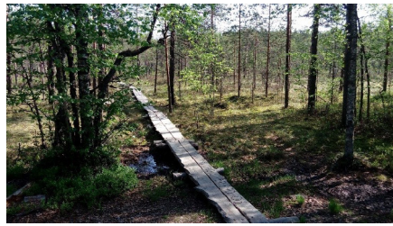
Figure 6. The walkway made of wooden boards.
