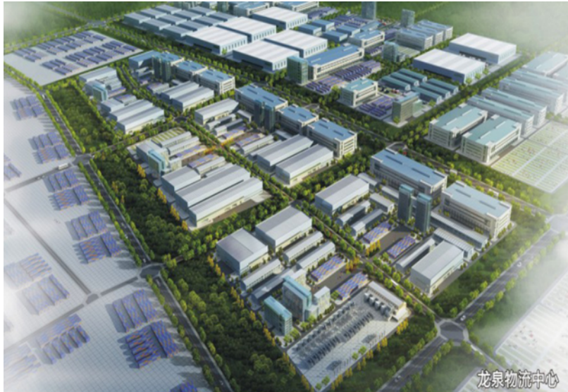
Figure 12: Chengdu Long Quan Logistics Centre(Source from: Chengdu City Planning Bureau 2016).
