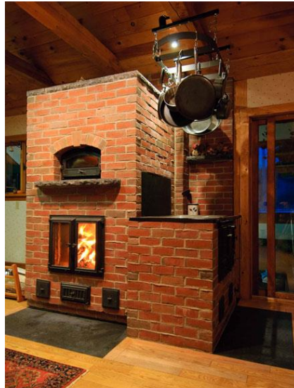
FIGURE 4. Masonry heater with oven /16/
