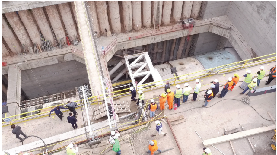
PICTURE 5. Sarmiento`s underground railroad renovations (Presidency of the Argentine Republic 2016).
