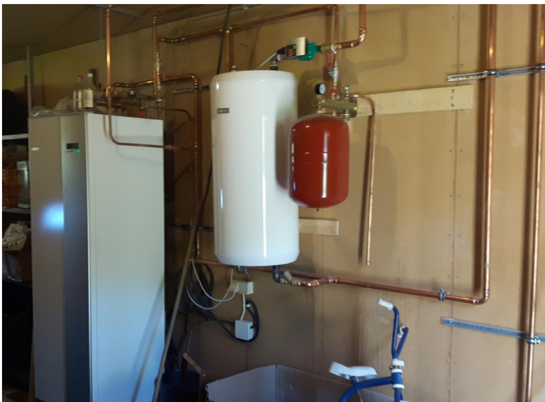
Figure 3-6. Nibe F1245, heat-pump unit. On the right side the Nibe UKV, next to the expansion vessel
