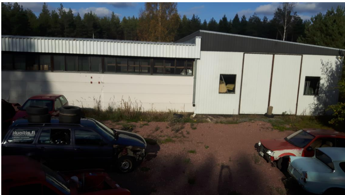
Figure 3-4. Other side of the mechanical shop construction
