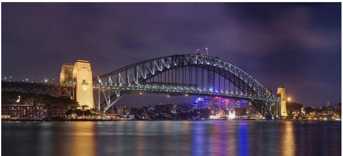
Figure 3. Sydney Harbor Bridge, Sydney, New South Wales, Australia (2010) (7)
