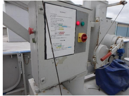
Green button on the side, main switch and brake lever
