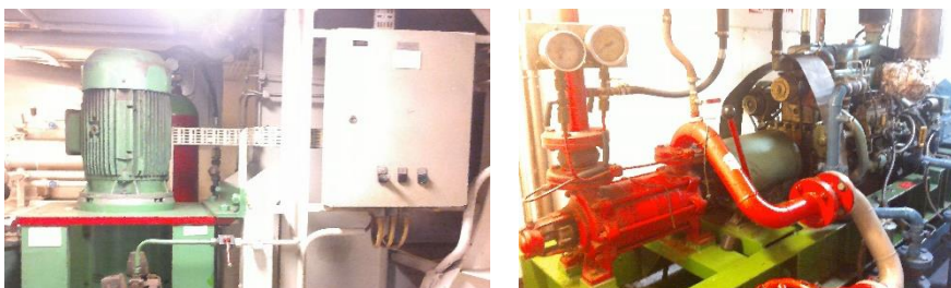
Ballast pump and switchpanel
