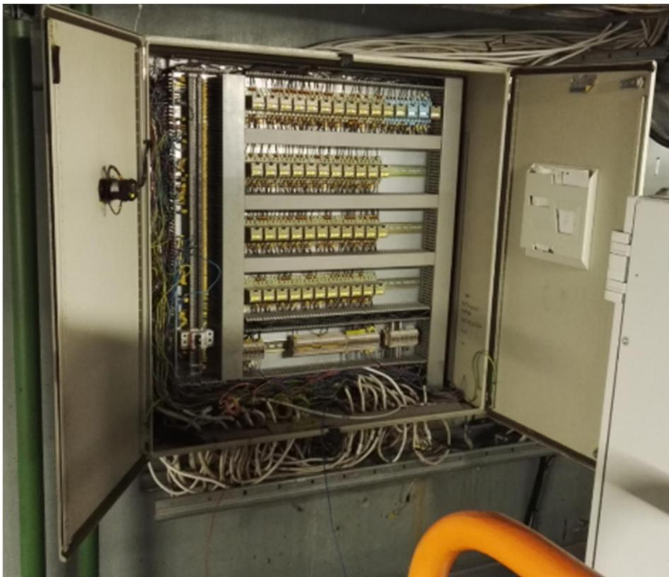
Figure 1. Common panel BAP903 messy and unclear wiring created by many modifications and add-ons.
