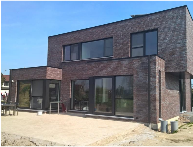
Figure 7. Massemen nZEB Photo 1
