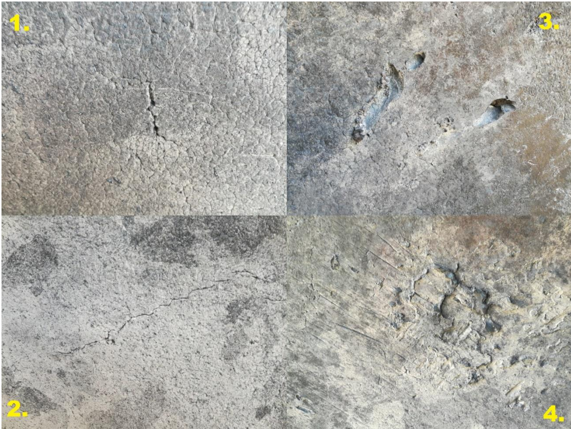
FIGURE 8. Different kinds of defects in the slag pot
