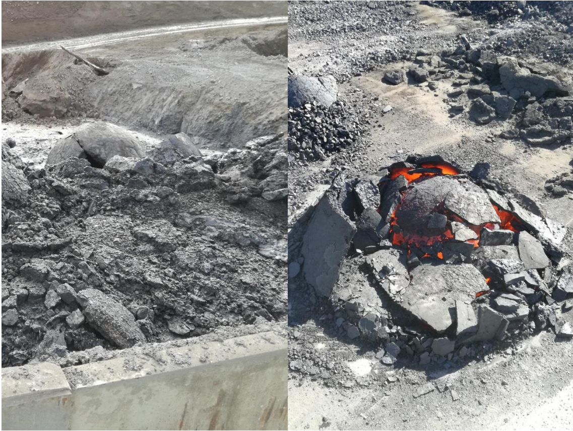
FIGURE 21. The natural sand has either been melted or pushed aside
