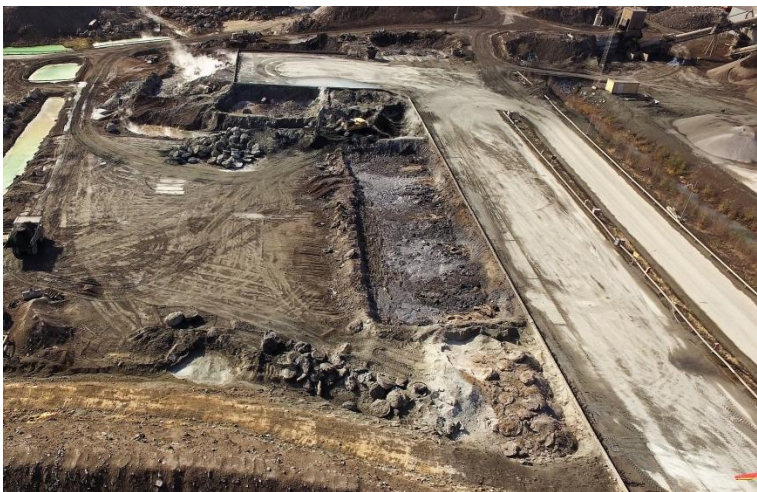
FIGURE 3. The dipping pits for the LD slag and the desulphurisation slags
