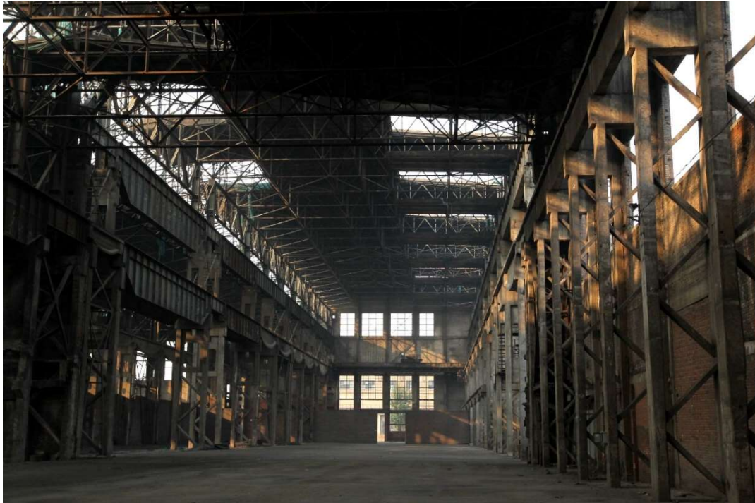
Figure 4.3. Old steel frame building in the US (40)
