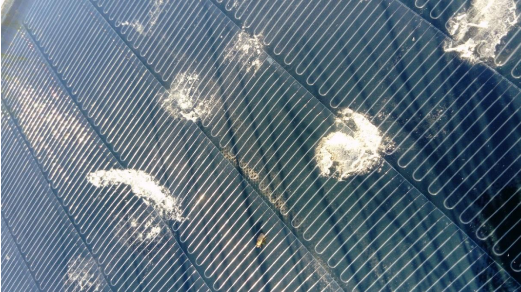
Picture 12. The broken barrier plastic and other damage
