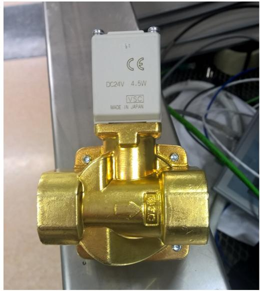
Figure 13. New magnetic valve (photograph taken by the author)
