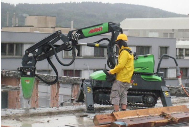
PICTURE 12. The operator is operating the demolition robot remotely. (Konepörssi. 2014.)
