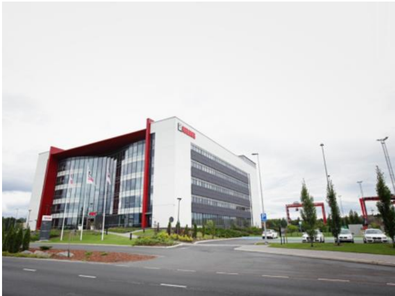
PICTURE 1. Cargotec Technology and Competence Centre in Tampere is one of the most energy efficient office buildings in Finland. (Cargotec 2018b)
