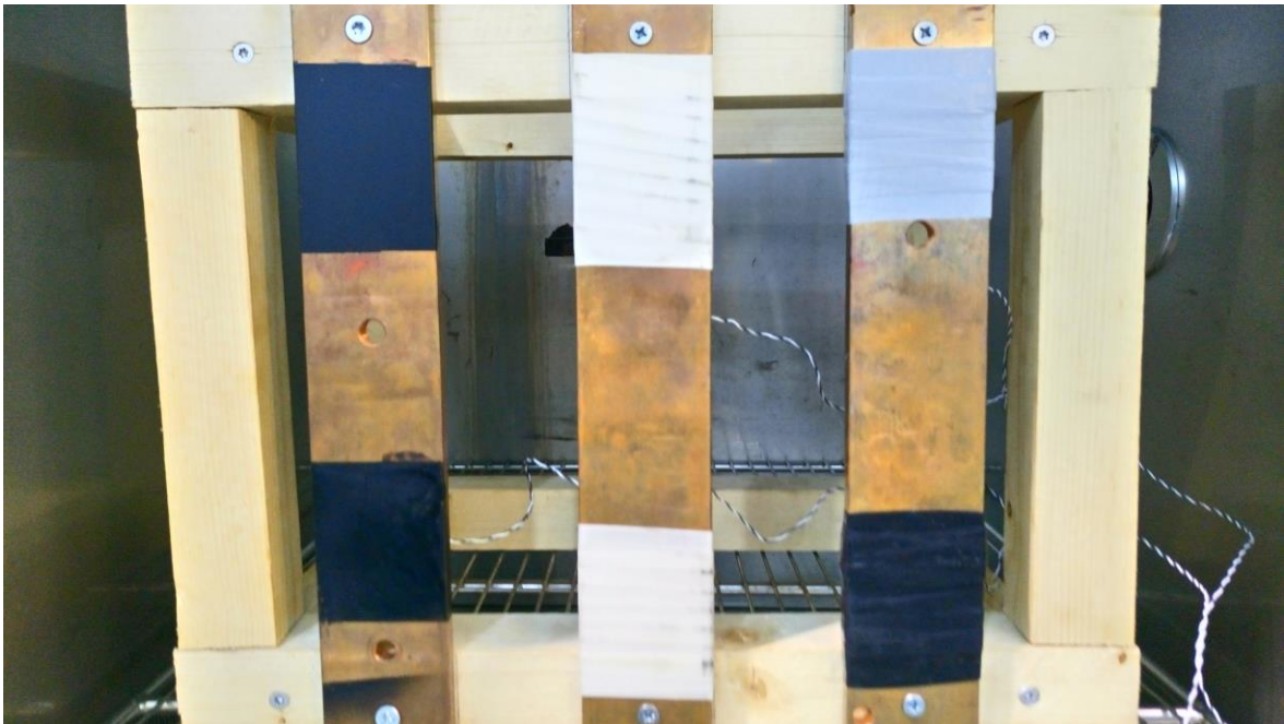
Figure 12 - The sensor's view of the bus bars
